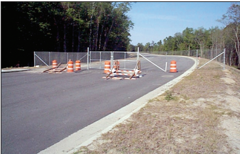
A spine road has been built through the megasite.
